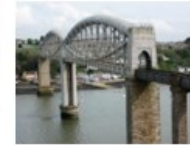
1859 - Royal Albert Bridge over River Tamar built. Designed by I K Brunel.
